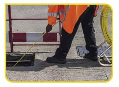
**2.** Feed the rod slowly into the conduit by hand, until the guide tip reaches the destination.
